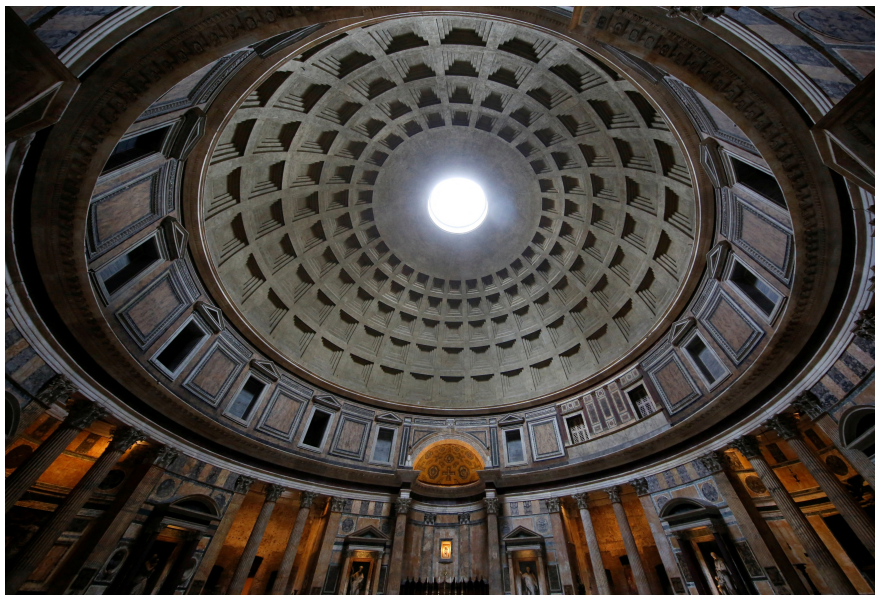
The Pantheon, Rome. After 2000 years, still the largest unreinforced concrete dome in the world.
