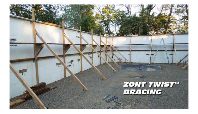
Bracing is critical on ICF construction, but when done correctly, and following proper pouring and consolidation techniques as recommended by the manufacturer, chances of a blowout can be eliminated. ICF specific bracing and scaffolding systems can often be rented from ICF dealers.
